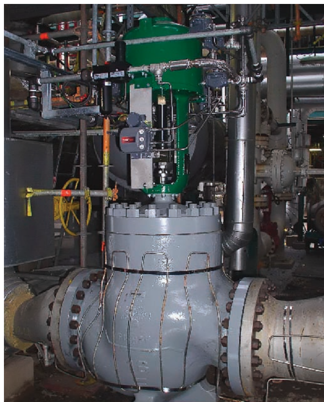
FIG. 3 This antisurge valve has been configured to meet the new performance criteria.
