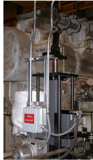
Figure 4. Electric Actuator direct on valve rack
