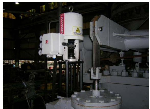
Figure 3. Pneumatic Actuator on pilot operator power cylinder
