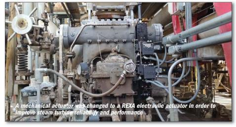
Controlling compressor efficiency starts with precision control of the ST driver in order to regulate the speed of the compressor. Actuator upgrades depend on turbine design.
